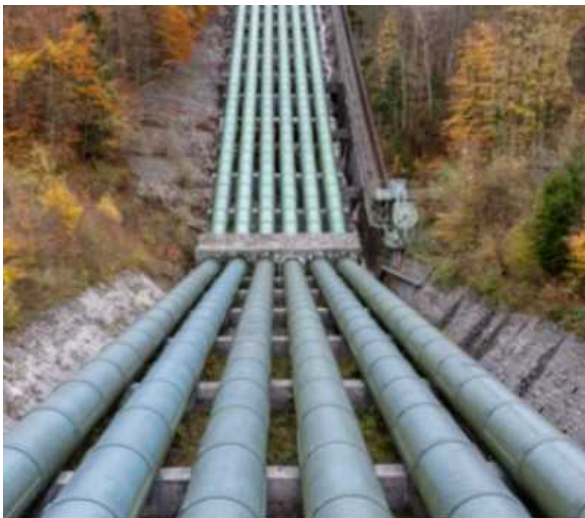
Gambar 38. pentstock Sumber : shutterstock
